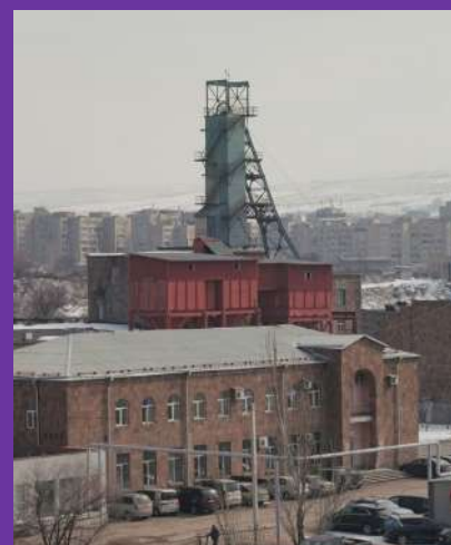
Avan Salt Plant Credit: Amos Chapple
